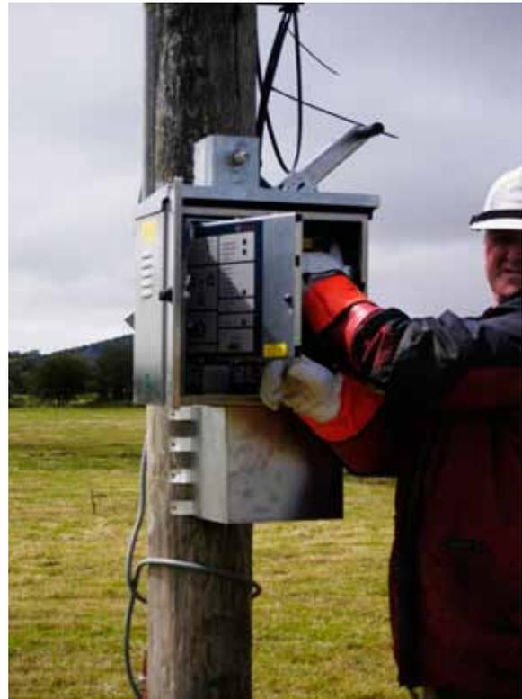
Where an Intelligent switchgear device is installed, such as a 'Smart Recloser', the data radio is connected to the device directly using a serial cable.
